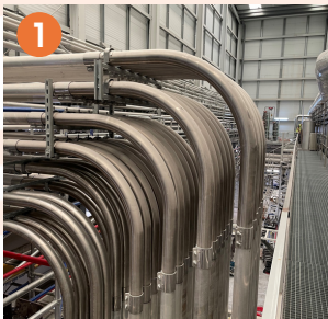
Material pipelines & accessories Pipe: Alu / SS / Flexibles / FU / PVC Elbows: SS / Anti-abrasive
