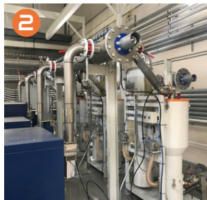
2 Central vacuum ring (energy saving)
