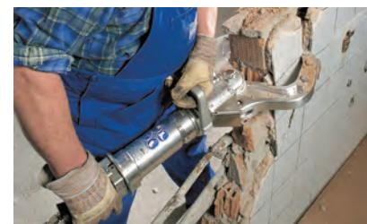
The HCS6 J is able to crush concrete walls up to 15 cm (5,9 inches) thick (depending on compression strength of the concrete). A big advantage for breaking, separating walls, facade or reclamation concrete panels.
