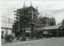
1968 • Delivered the industry's first supercritical pressure boiler, Chubu Electric Power Chita No. 3 (1,700t/h)
