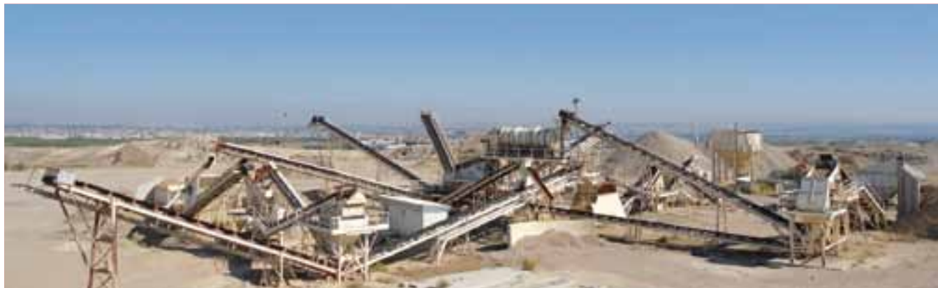
PRIMARIO - ARJA TAURO 25 & TUSA HN45 SECUNDARIO - ARJA PISCIS 2000 & TUSA HN60 LAVADO - TUSA HN60 & TSL100, 200Ton / HOUR – Ubicado en / Located in Vertedero Las Canteras, Zaragoza CONTACT: Ramon Calvet, (+34) 667.004.472
