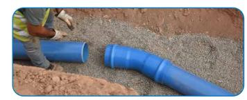
During assembly, avoid blows to the fitting, especially on the groove of the socket joint, recommending its manual installation whenever possible or the use of cloth slings.
