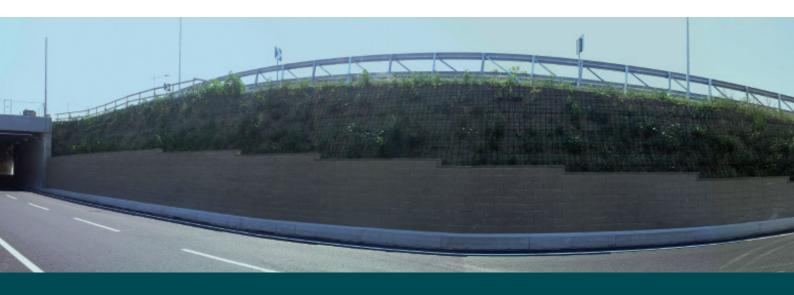
The innovative MacWall system was invented to cater for the increasing demand for high-tech containment structures and retaining walls with reduced labour costs and fast construction times. The high level of design flexibility and in-depth analysis of the various components produced a rapid, economical, modular, versatile, green and innovative system
