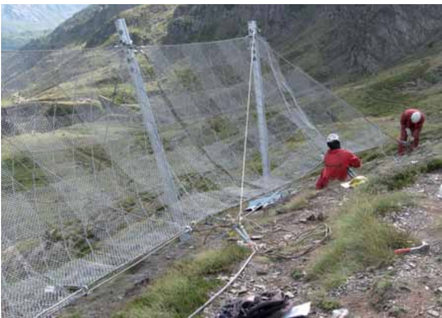
Installation of pre-assembled units delivered by helicopter
