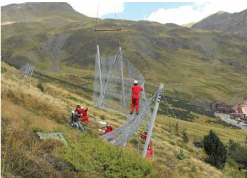
Installation of pre-assembled units delivered by helicopter
