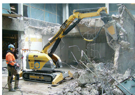
Crusher with additional teeth
