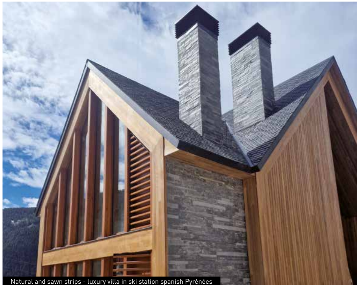
Natural and sawn strips - luxury villa in ski station spanish Pyrénées
