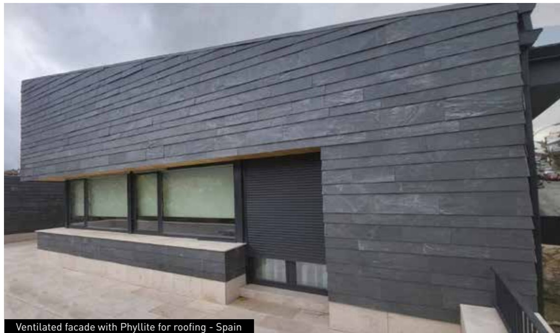
Ventilated facade with Phyllite for roofing - Spain
