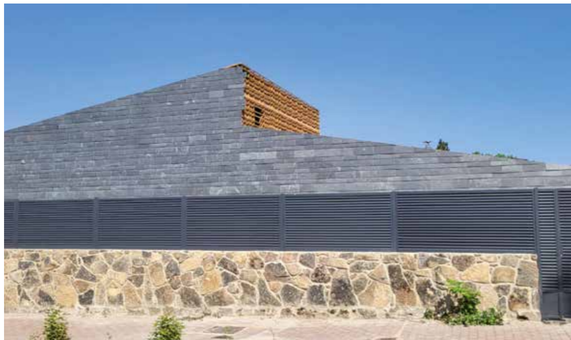
Ventilated facade with Phyllite for roofing - Spain
