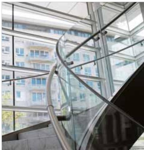
For straight handrails, changes of direction can be handled in one of three ways. Handrail components with 45 and 90 degree bends are available as standard items, ready to cut to length during installation. For other angles you can either form a bend in the rail or use the unique Omnibend component, which can be easily adjusted to any angle on site.
