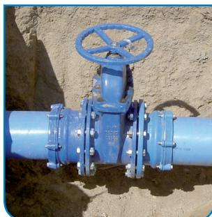
Anti-traction system makes the pipe absolutely fixed to the flange.
