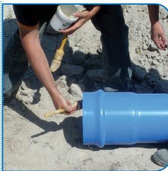
Apply lubricant on the chamfer of the spigot end and in the rubber ring joint.
