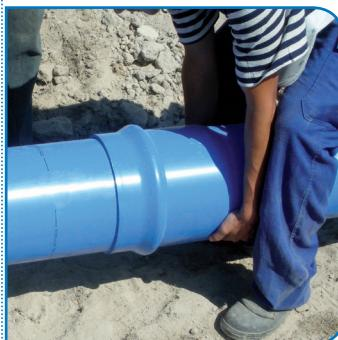
Align the pipe and place the spigot end inside the socket or bell.
