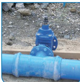
It is very important to fix the fitting to the ground in order to guaranty the net structural resistance.
