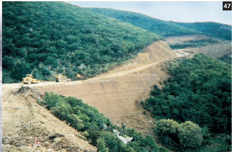
47-48. Road embankment using geogrids and Green Terramesh® mixed structure, Villamassargia (CA)-Italy.
