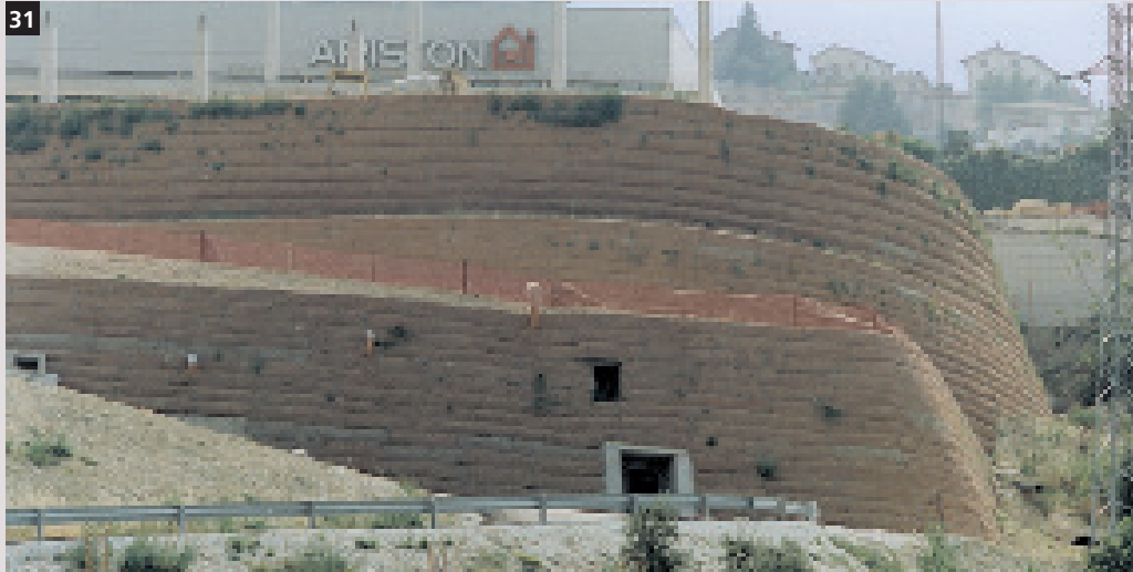
31, 32. Retaining structure in Green Terramesh® to extend industrial building, Arcevia (AN)-Italy.
