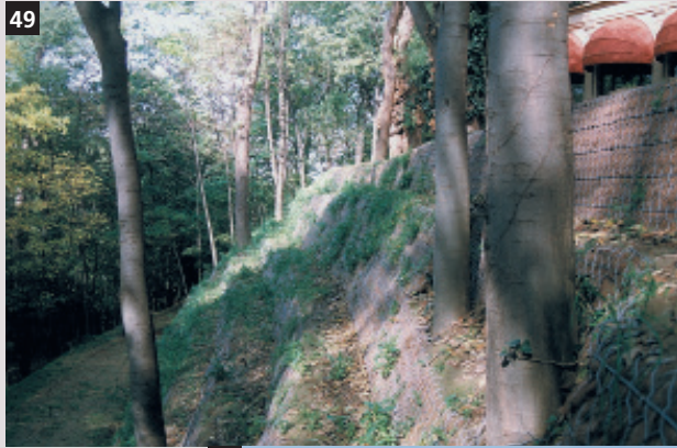
49. Green Terramesh® retaining structure, Bologna-Italy.
