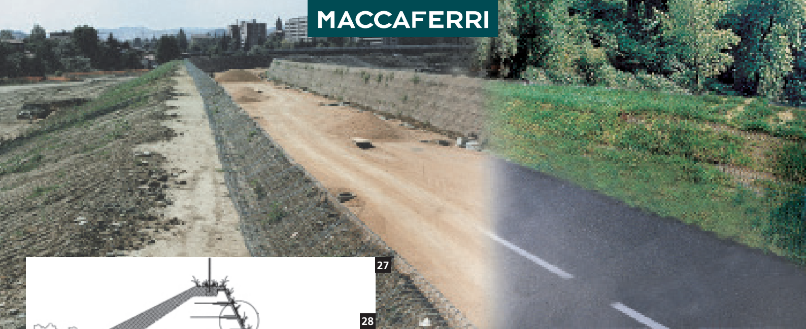
27-28. Green Terramesh® sound barrier in urban area, Bologna-Italy.
