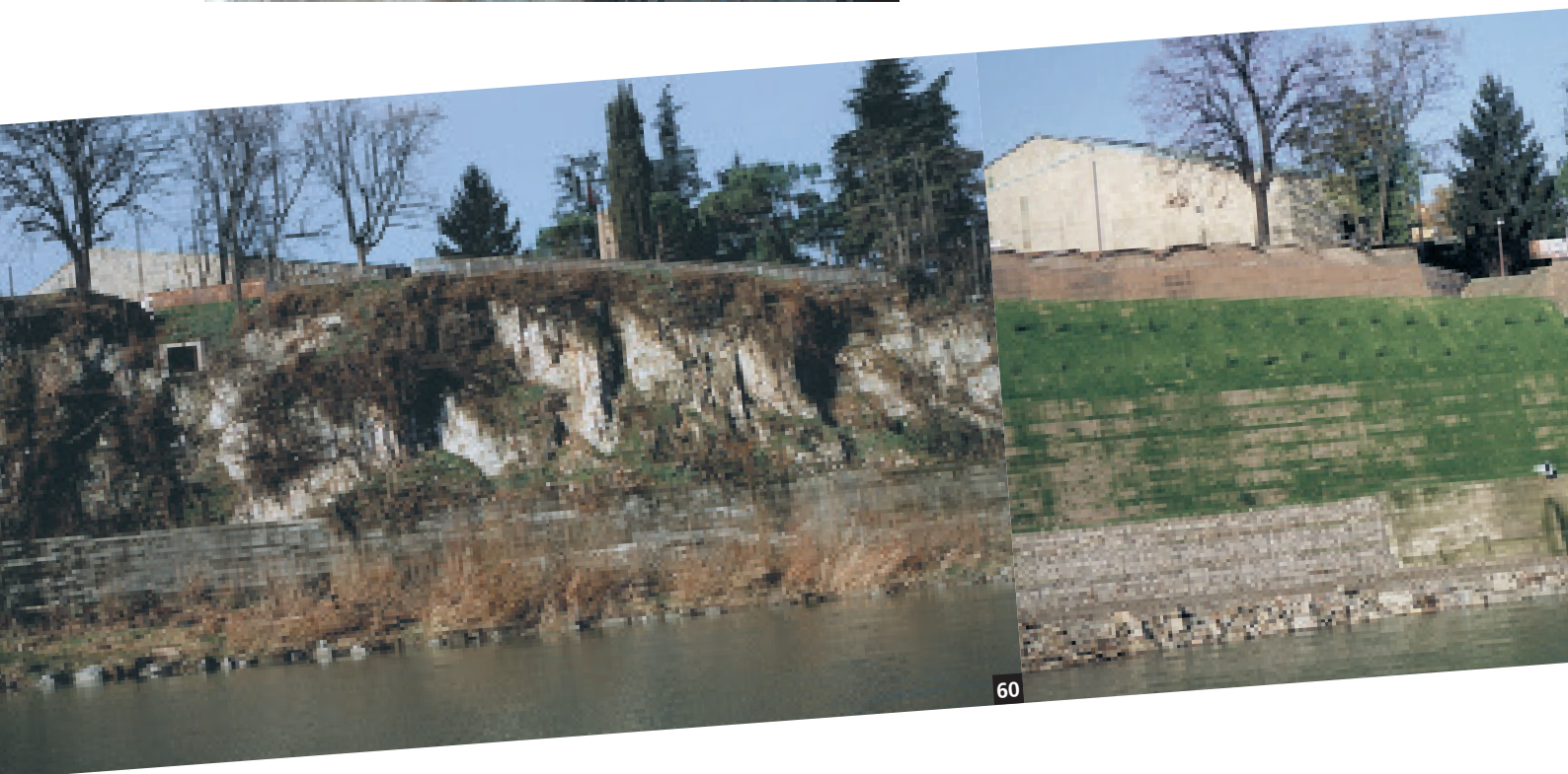
60-61-62. River bank protection for environmental rearrangement and the construction of a cycle footstep using Terramesh, Casalecchio di Reno (BO)-Italy.
