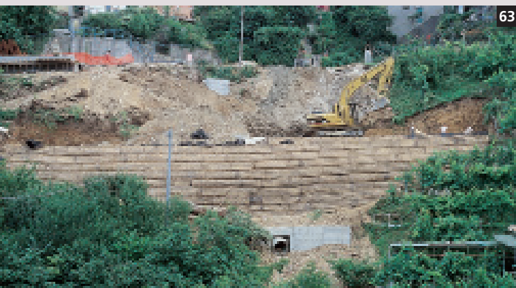
63. Geogrids retaining structure for enlargement of a road, Arcola (SP)-Italy.
