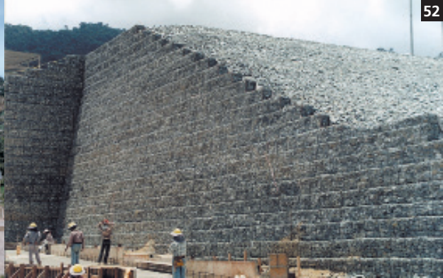
50. Retaining wall for new parking area with Green Terramesh®, Ariccia (RM)-Italy.
