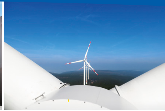
© Vensys 112, 2,5 MW, Wind farm in Losheim-Britten, Germany
